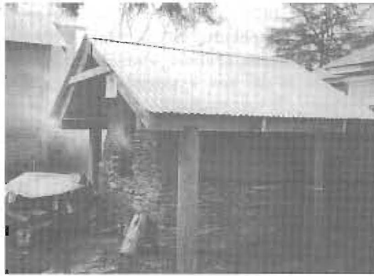
FIGURE 9. The reconstructed Ratto oven, behind the Calaveras County Historical Society Museum in San Andreas; photographed in 1995.
