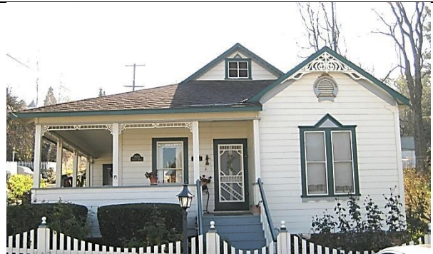
Bennett House, No 37 (c. 1890)
