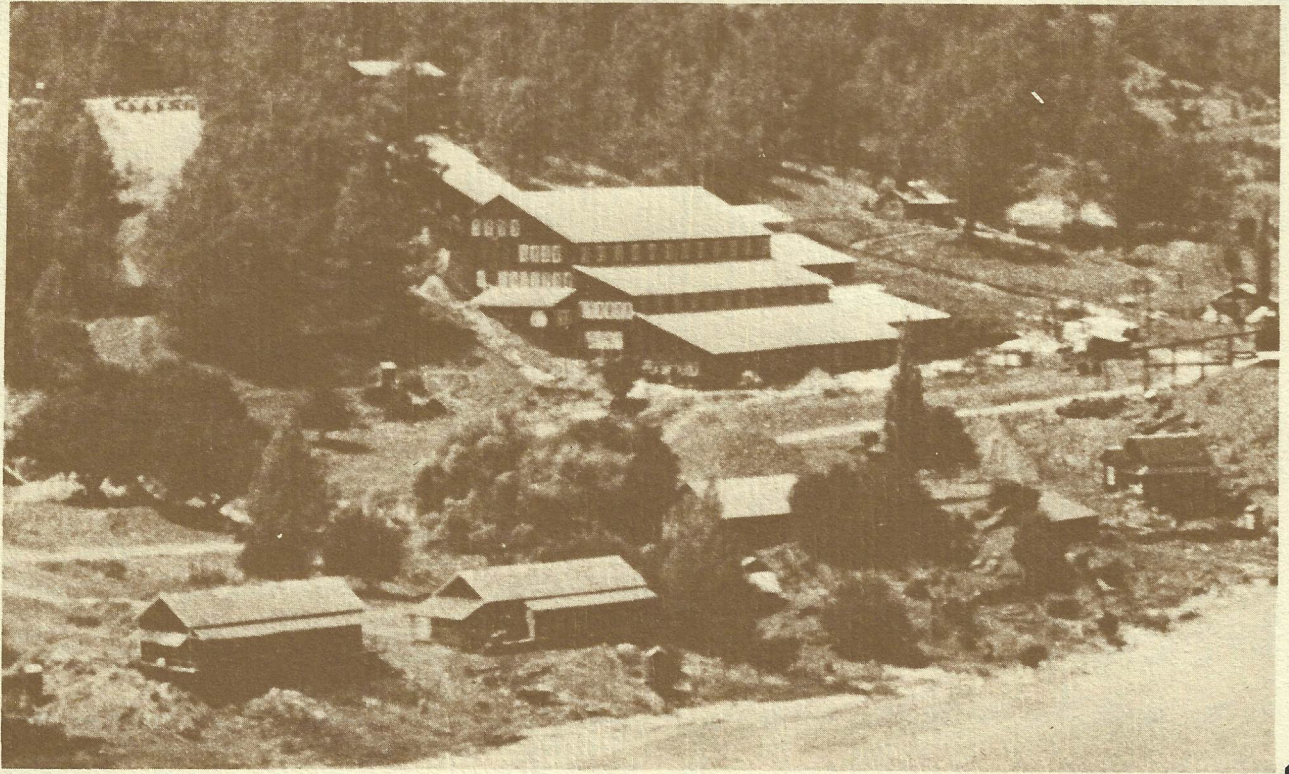
Figure 27: The mill of the Melones Mining Company constructed in 1902 with sixty stamps and enlarged to one hundred stamps by 1906. The white rock dump from the Melones adit is seen to the upper left and in the foreground are bunkhouses for the miners. Courtesy of the Calaveras County Historical Society.
